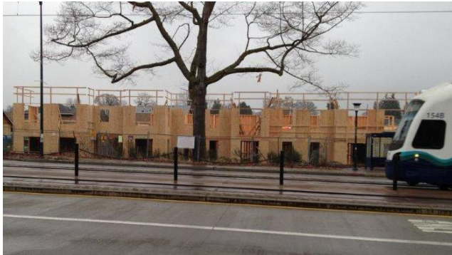
Columbia City Station Apartments: 52 units of new, affordable workforce housing with a “live/ work/ play” design, located at a transit and pedestrian oriented site.
