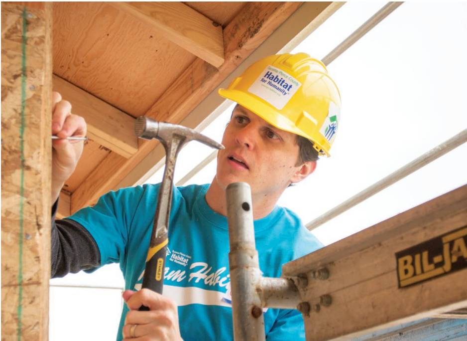
A Habitat volunteer helps build a home in Pierce County.
