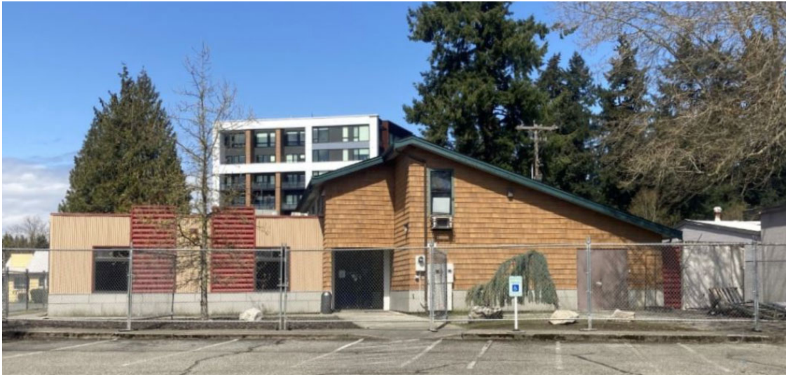
The former dog daycare, now demolished, at 16725 Cleveland Street would become 100 units of housing available to people with disabilities who are directly exiting homelessness under Redmond’s new plan. (City of Redmond)
