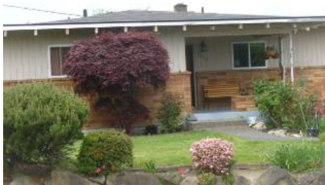
The exterior walls are partial brick veneer and wood.
