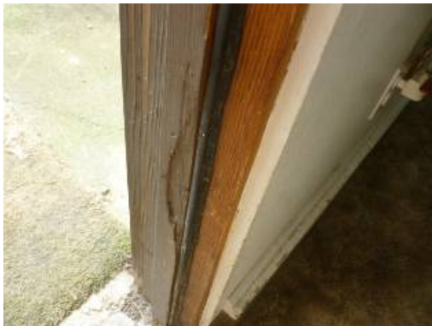
Upgrade weather stripping on doors.
