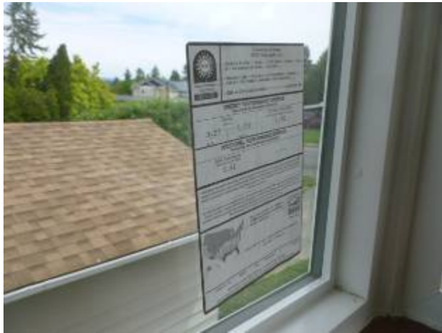
Almost every window has been upgraded.
