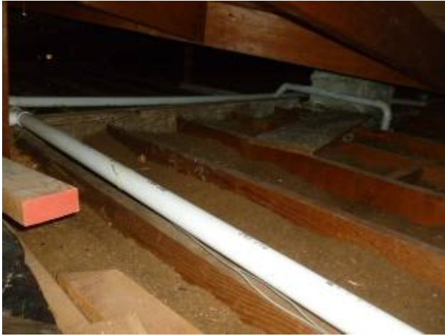
Add cellulose insulation on top of the old silva wool.
