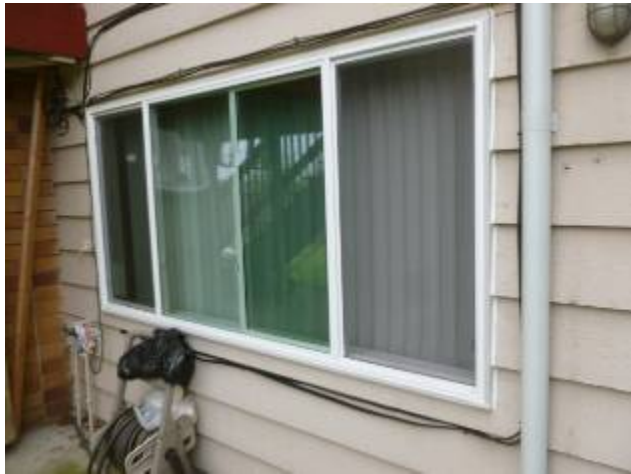
Basement walls have horizontal siding.
