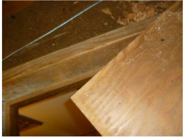
Weather strip and insulate the attic hatch.
